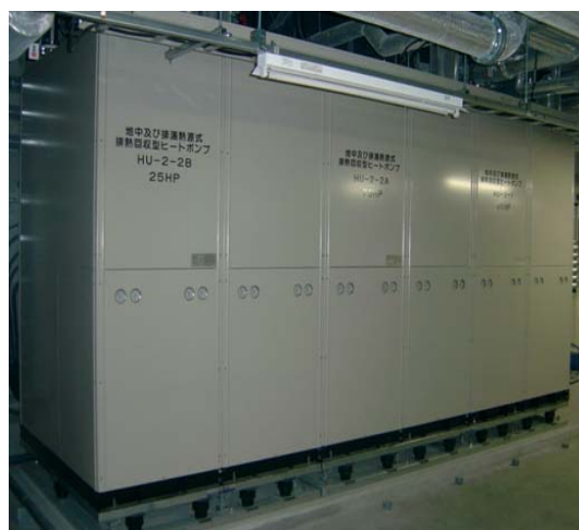
Figure 4 Water-to-Water Heat Pumps
